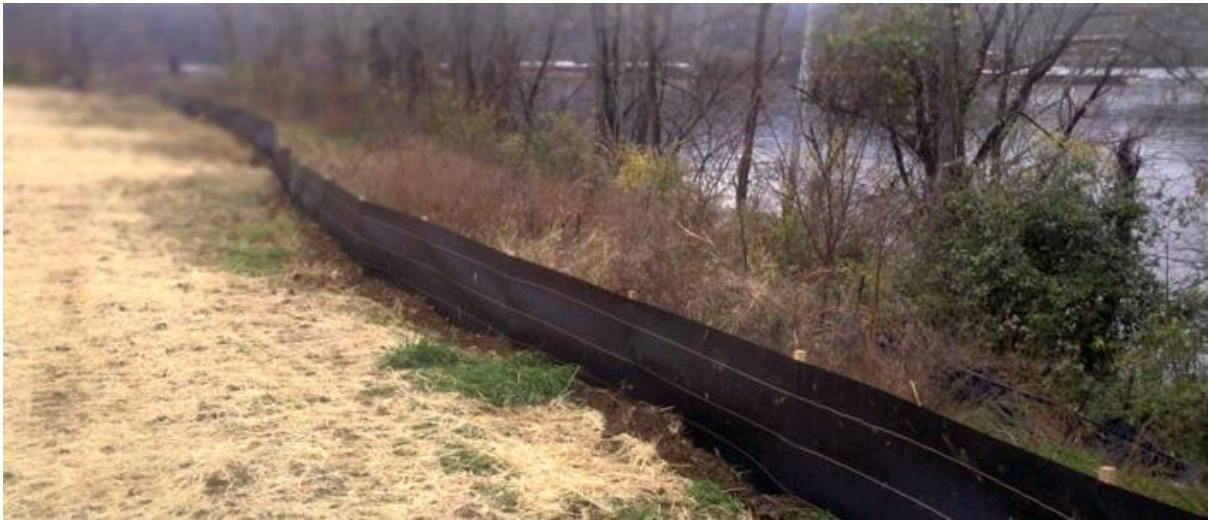
Figure 10-4 Silt Fence Installed alongside Riverbank [Source Thrace Synthetic]
